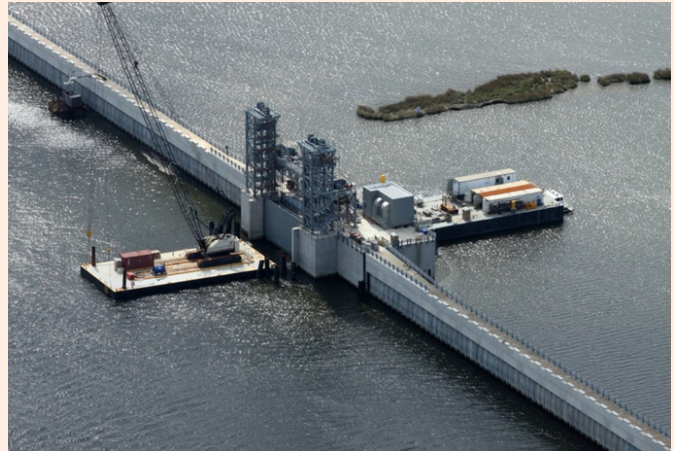
Lake Borgne Surge Barrier gate. Source: U.S. Army Corps of Engineers
