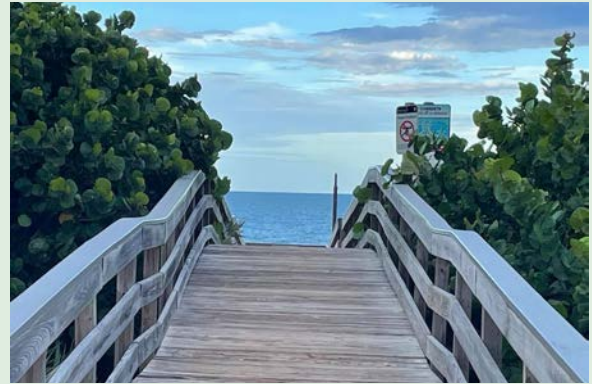
Dune crossover structure at Canaveral National Seashore. Source: Florida Today
