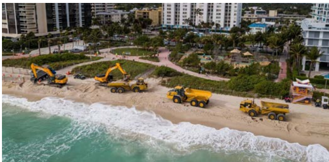
Beach renourishment activities. Source: Matais J. Ocner | Miami Herald
