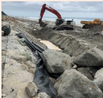
Buried revetment acting as the last line of defense at Cardiff State Beach. Source: City of Encinitas.
