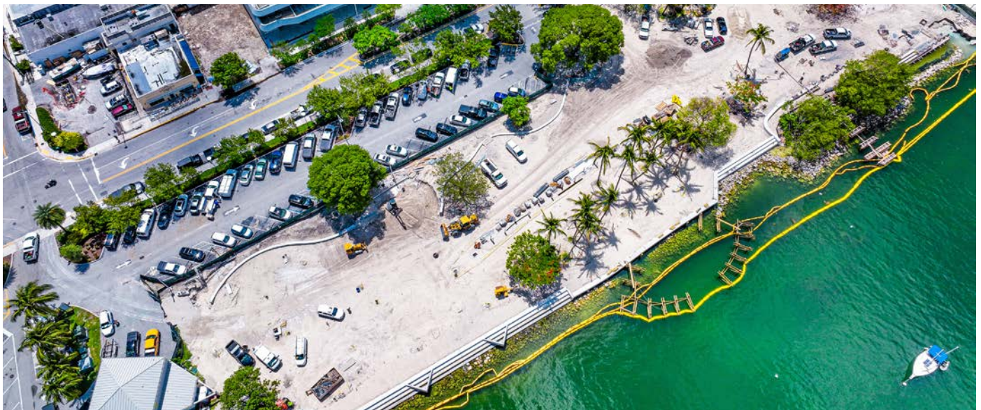
Aerial view of construction at Maurice Gibb Park. Source: Miami Beach
