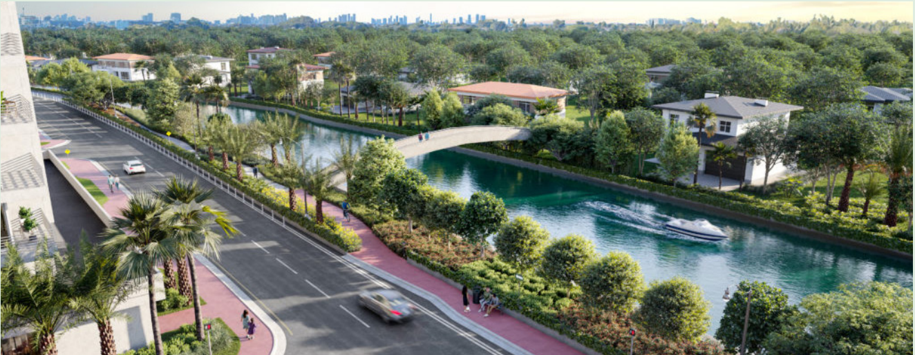
Use of blue-green stormwater infrastructure elements at Canopy Park. Source: Miami Beach
