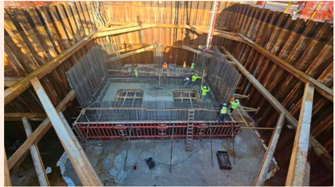
West Avenue Pump Station under construction. Source: Miami Beach
