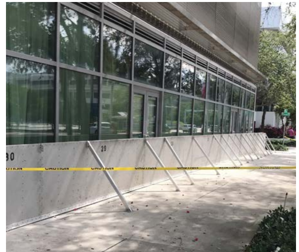
Use of flood barriers to protect building from flood damage on Pennsylvania Ave. Miami Beach. Source: Miami Beach
