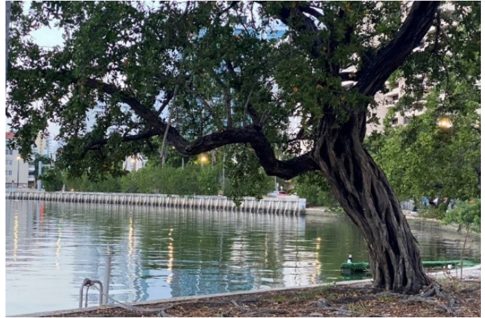
Seawall upgrades at Parkview Island Park, Source: AECOM
