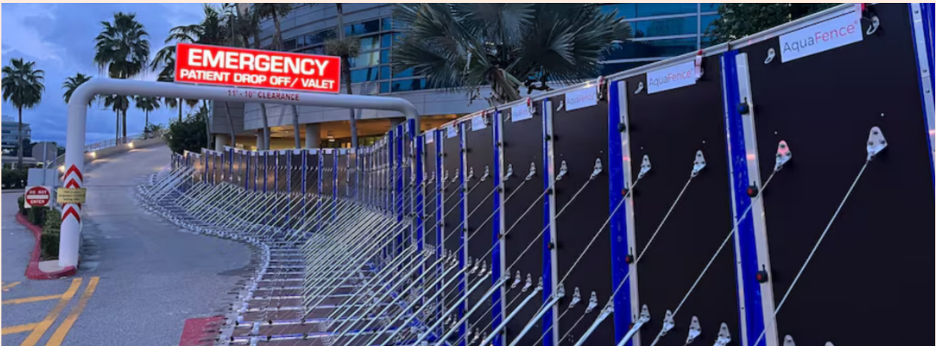
AquaFence flood barrier at Tampa General Hospital ahead of Hurricane Ian (Sept 2024). Source: Tampa Bay Times
