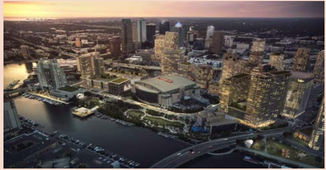
50-acre redevelopment on Water Street in downtown Tampa featuring waterfront setbacks that began in 2017. Source: Water Street Tampa
