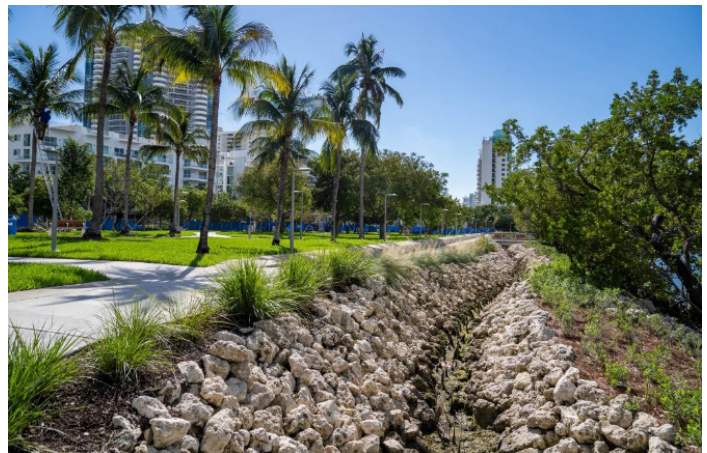
Living shoreline installation at Brittany Bay Park, Source: Miami Beach
