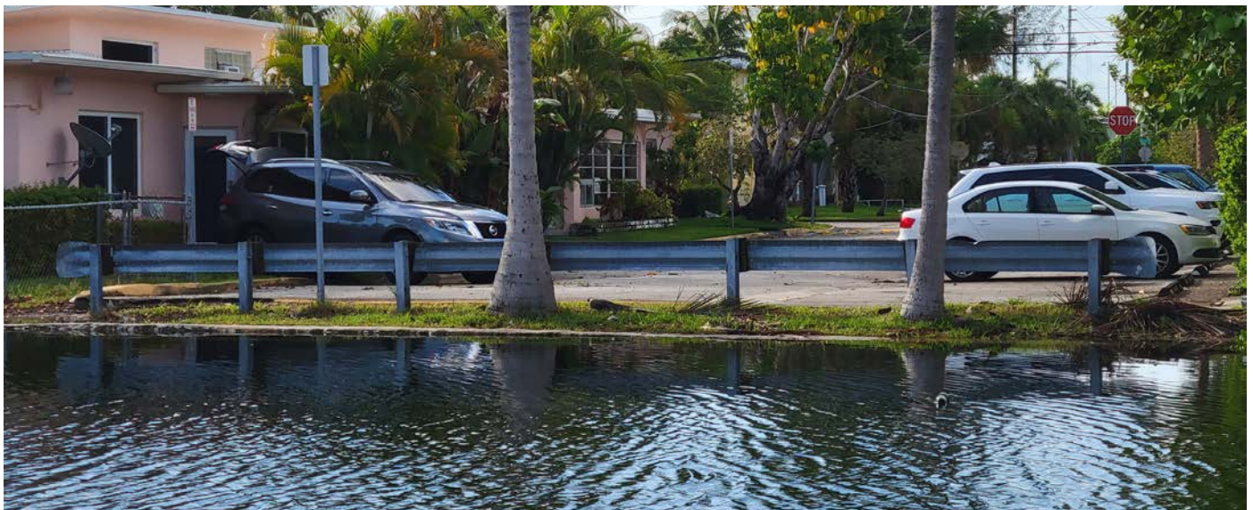
Miami Beach canal seawall overtopped during king tide event. Source: Miami Beach
