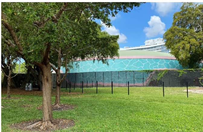
City drinking water storage tank, Source: AECOM
