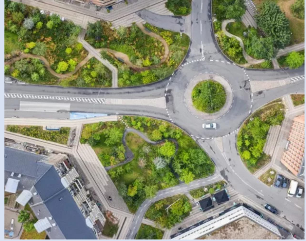
Sankt Kjeld's Square & Bryggervangen pilot road detention project, Copenhagen, Denmark. Source: SLA
