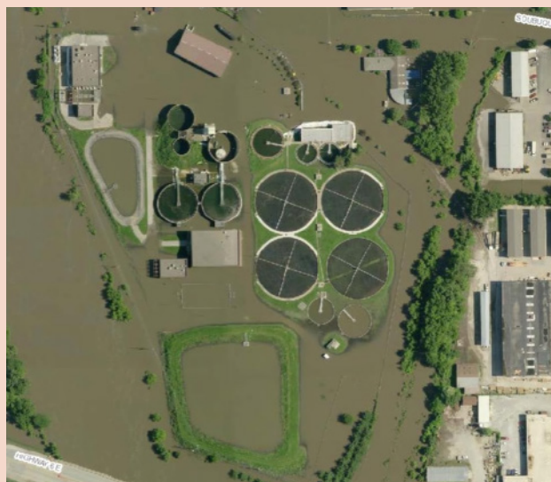
Flooded North Wastewater Treatment Plant.
