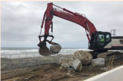
Buried revetment acting as the last line of defense at Cardiff State Beach. Source: City of Encinitas.
