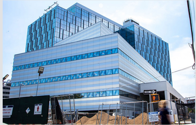
The Ruth Bader Ginsberg Hospital constructed with FEMA funding following Hurricane Sandy, New York City. Source: The City of New York
